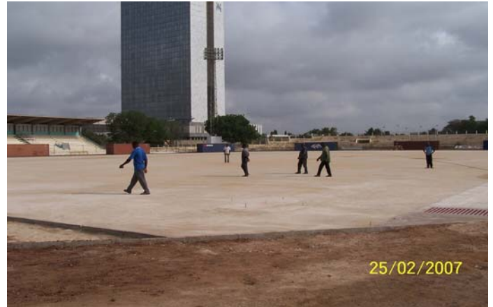
Preparation work for the new football turf pitch.
