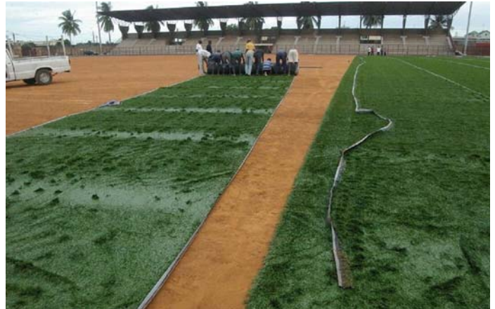
United manpowers installing the new football turf.
