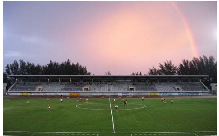
The same stadium after installation of a FIFA-approved football turf pitch. Costs were born 50-50 by FIFA and the Seychelles government.
