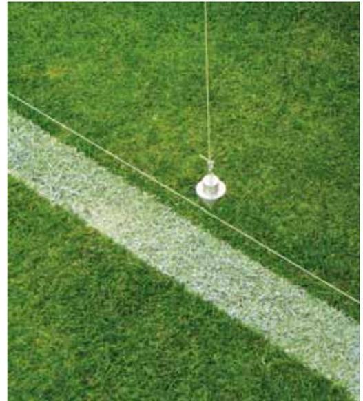
Final installation test – dropping a plumb to define the goal line
