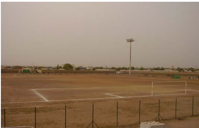
The Stade Gouled, Djibouti prior to the start of renovation work.
