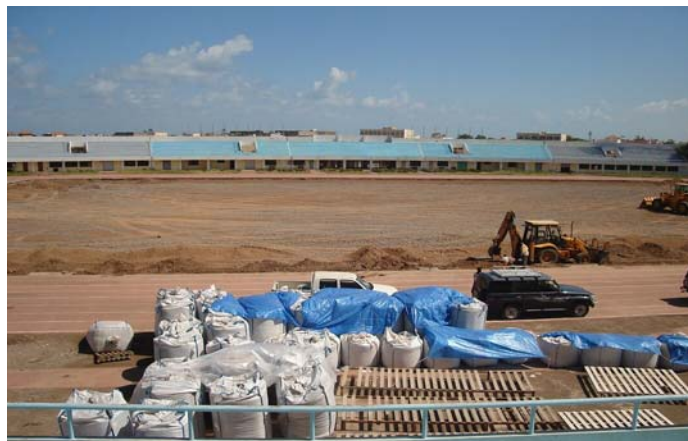
Installation of a full-size football turf pitch in 2007.
